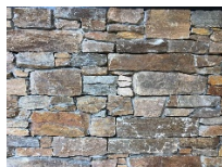
Figure 1.5 BlueStone cladding to masonry.
