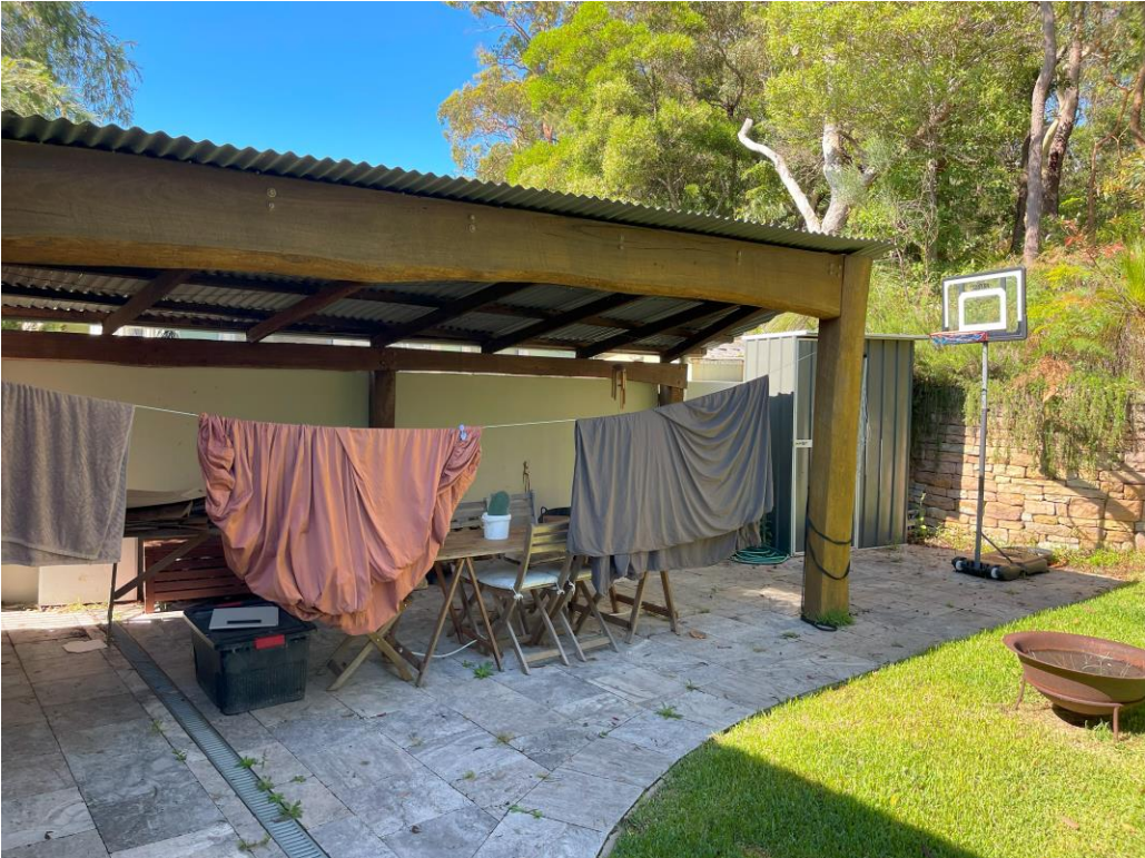
Fig 7: View of the patio area, looking south-west
