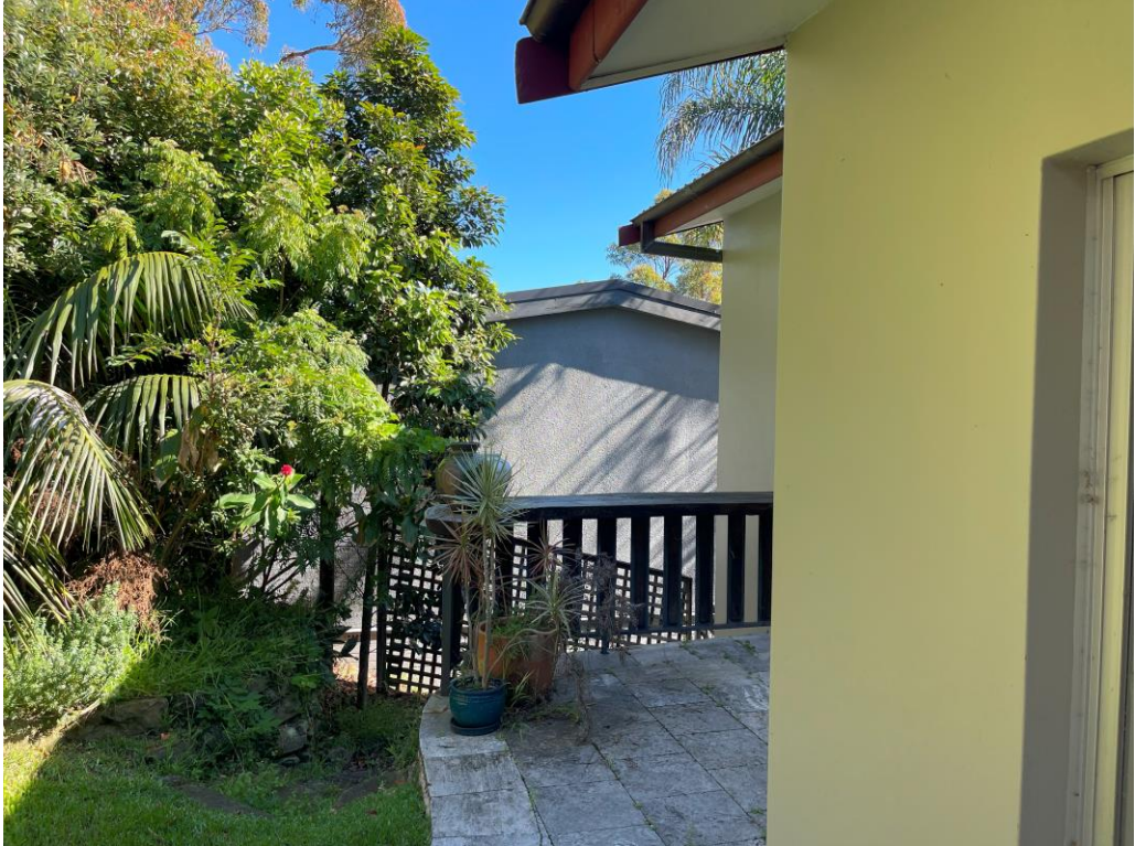
Fig 6: View looking north across the rear façade of the dwelling
