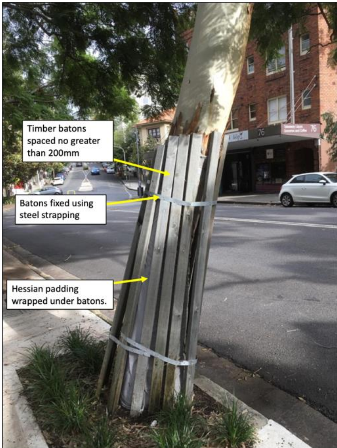
Figure 10. Example of properly installed stem protections measures.
