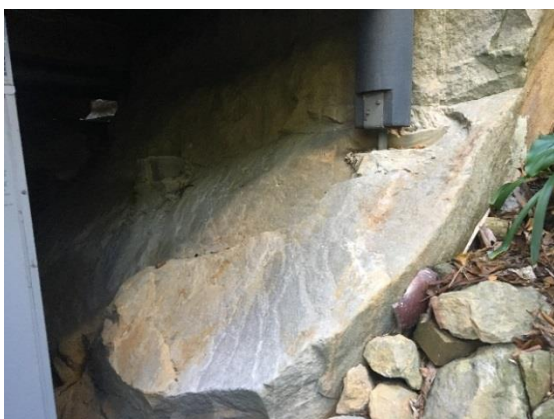
Photo: 7 - House supported off boulder
