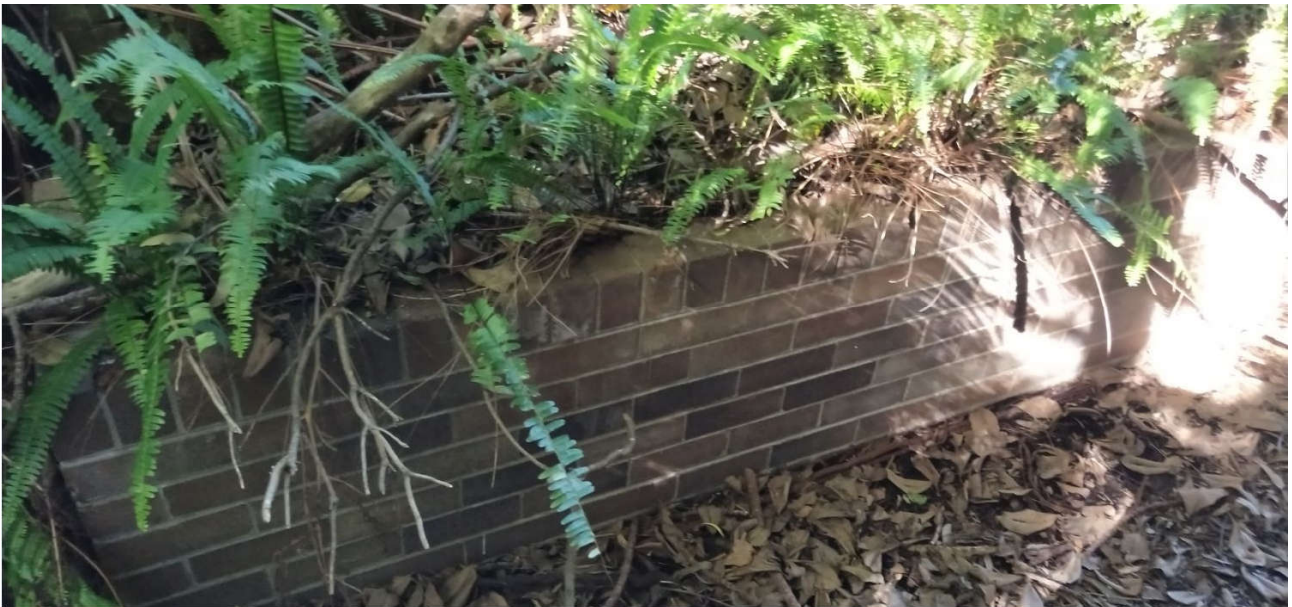
Plate 2: Photograph of 0.7m High Brick Wall Assessed to be in Poor Condition
