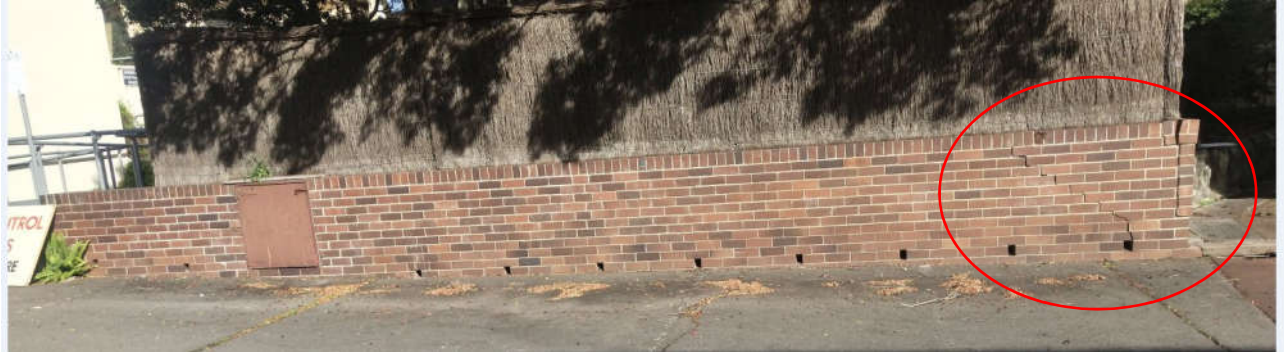
Plate 2: Photograph of 0.7m High Brick Wall Assessed to be in Poor Condition
