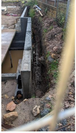
Cut face on adjoining site with retaining wall, prior to backfill
