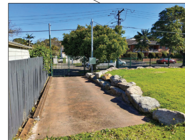
EXISTING HARDSTAND ALONG NEIGHBOURING PROPERTY TO BE DEMOLISHED AND GATE TO BE RELOCATED TO THE NEW EGRESS
