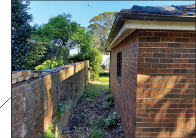
EXISTING BRICK MASONRY ALONG EASTERN BOUNDARY TO BE RETAINED AND REPAIRED FOR REUSE
