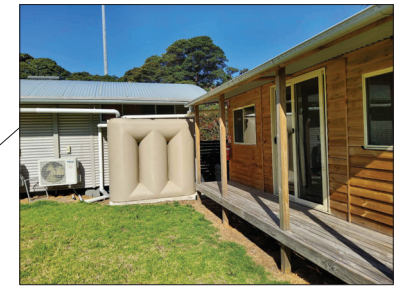
EXISTING STRUCTURE TO BE RELOCATED
