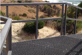
4. MARINE GRADE FRP MINI MESH WITH > 40% TRANSPARENCY FOR ALL TRAFFICABLE SURFACES
