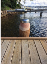
4. 300 DIAMETER TURPENTINE PILES WITH STAINLESS STEEL RINGS & CAPPING
