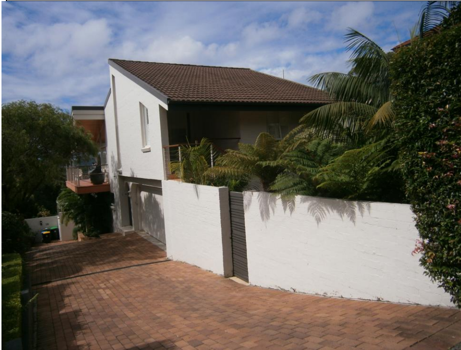
View looking down the driveway. Existing roof to be squared off to allow for an upper floor addition
