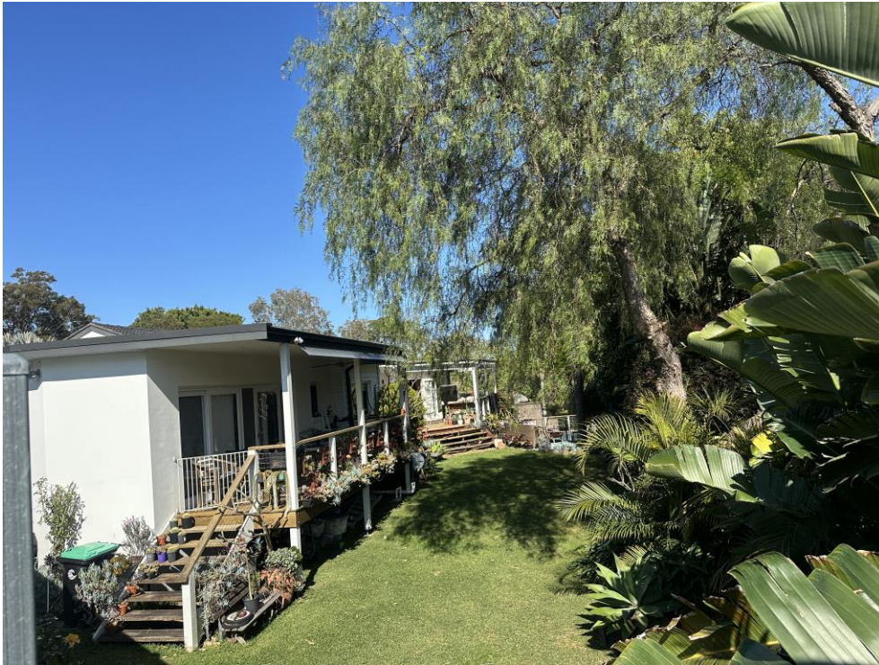
Figure 10. The existing secondary dwelling, looking north-east.
