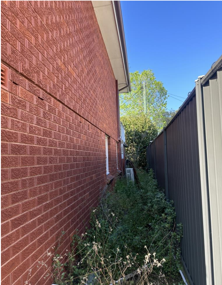
Figure 8. The west side boundary, looking south.
