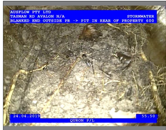
Photo: 3_1_17_24042019_133342_A.JPG 55.5m, A Mass of mostly fine Roots, which has developed into an interwoven clump , Obstruction: 21-50% , from 4 to 8 o'clock
