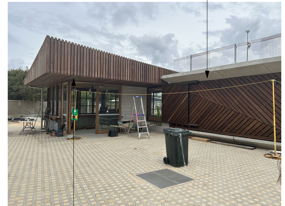
EXISTING TIMBER CLAD EAVE OVER TENANCY
