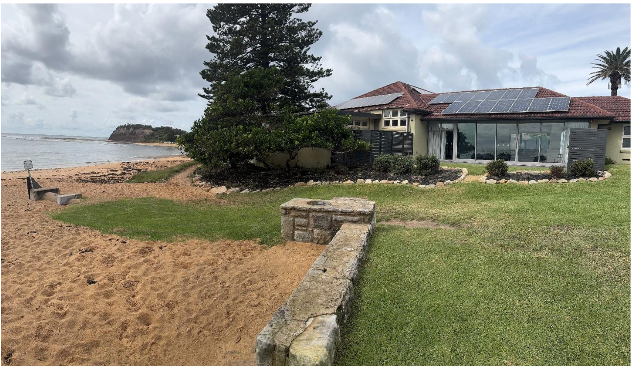
Photo 5 - The Site Looking East with the Stormwater Pipe at the Western Side of the Existing Building, 27 March 2025
