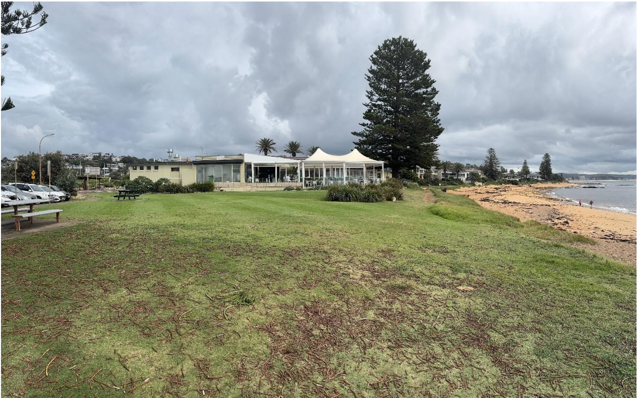
Photo 2 – The Site Looking West, 27 March 2025
