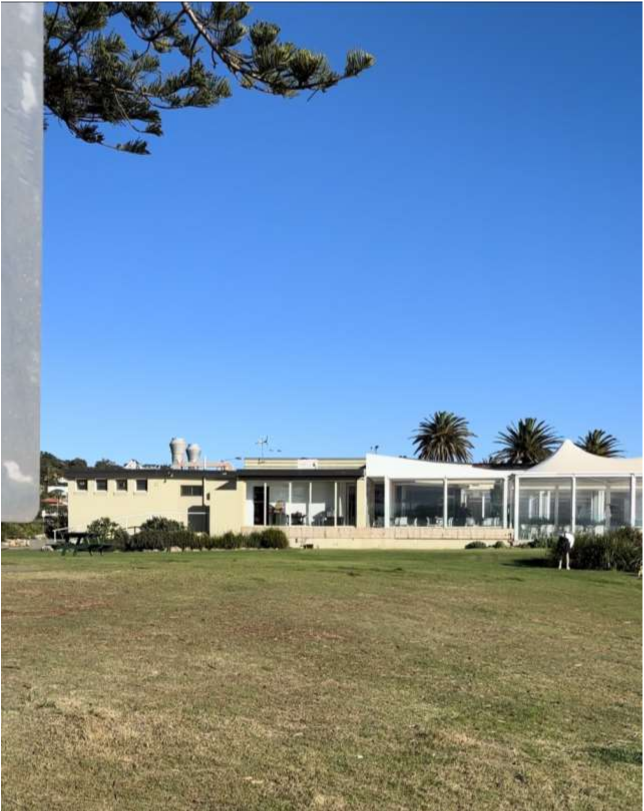
Image 4 – Existing Golf Clubhouse
