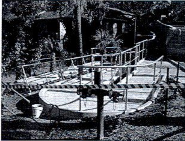
Accessibility ramp regarded with level 180 ° switch back max grade 1:14, 75 mm kerb and handrail to full length
