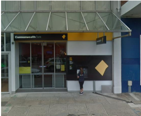
Photo 1: Existing Commonwealth Bank, Brookvale
