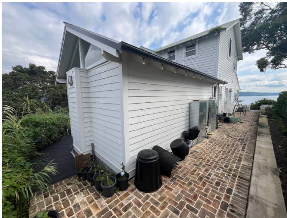
Photo 9: South western corner of the house
