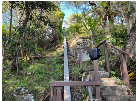
Photo 4: Inclinator access from site frontage to house, with outcropping sandstone bedrock and boulders along the path of travel
