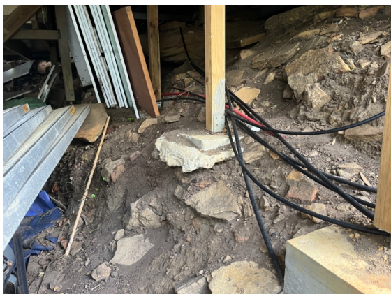
Photo 11: Example of footings on fill under the rear of the house
