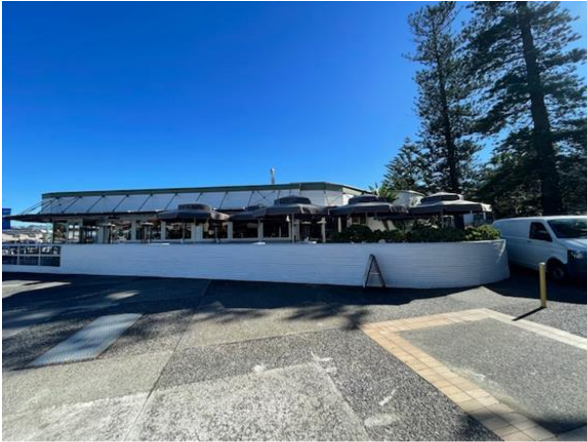
Figure 15: View facing east of the existing deck of Manly Wharf Hotel to be extended.
