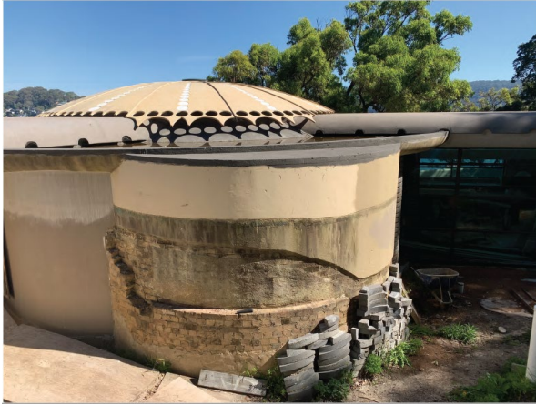
Figure 2 Detail of rear façade of sitting room.
