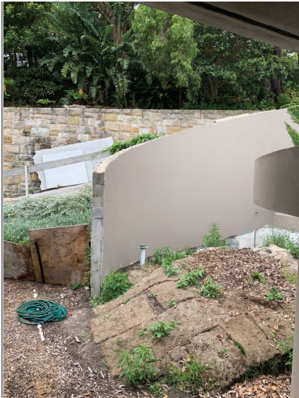
Figure 4 View of existing curved garden wall.
