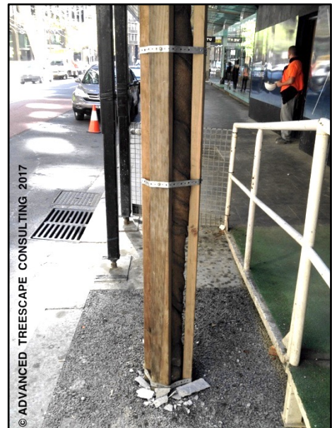
Example of Trunk Armour
