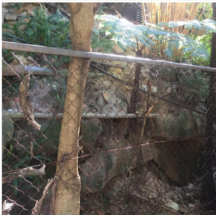
Embankment where the dispersion pit is planned to go. Stormwater from this has the potential to erode this bank and adversely affect the neighbouring property. Water can also seep into the neighbouring property and cause stability problems and dampness to beneath the neighbouring property.
