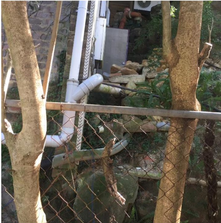
Stormwater pipes from subject property downpipes that flow to the extreme South West corner of subject block and discharge into neighbouring properties.
