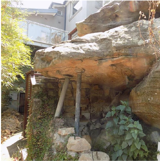
View of existing rock outcrop, stabilisation work and location of the proposed pool.
