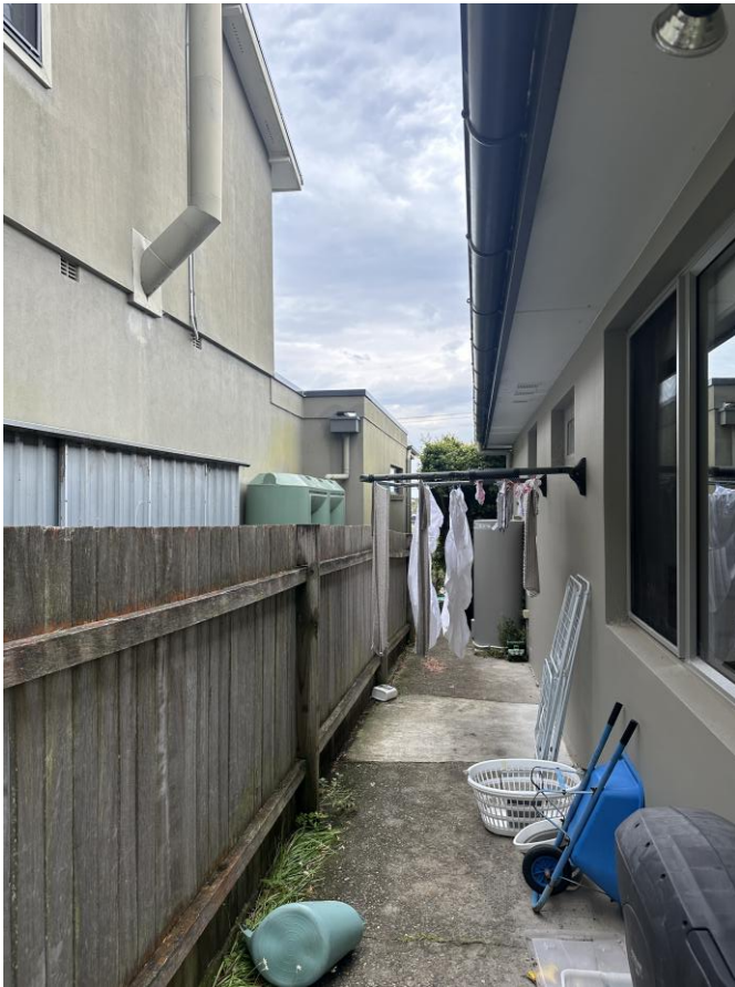
Figure 8. The northern boundary, looking east.
