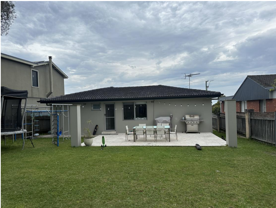
Figure 7. The rear of the dwelling, looking east.
