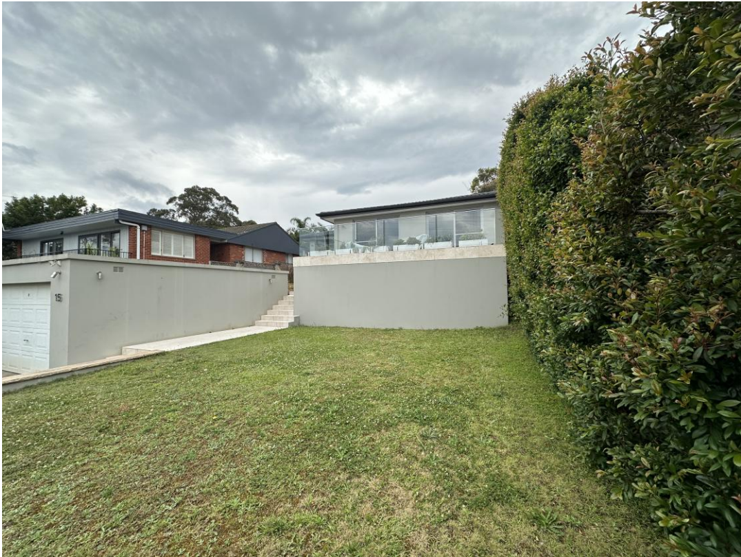
Figure 6. The front façade and existing front yard, looking west.
