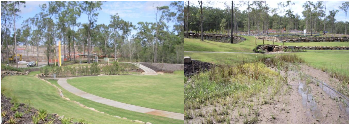
Figure 8-9 Example biofiltration basin integrated within community park (source: Lake Macquarie City Council, 2013)
