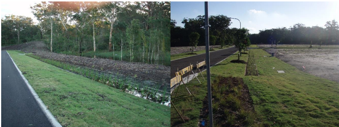
Figure 7-5 Grassed roadside filter strips
