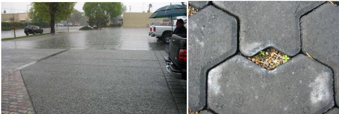
Figure 7-4 Pervious concrete (LHS) and permeable pavers (RHS)
