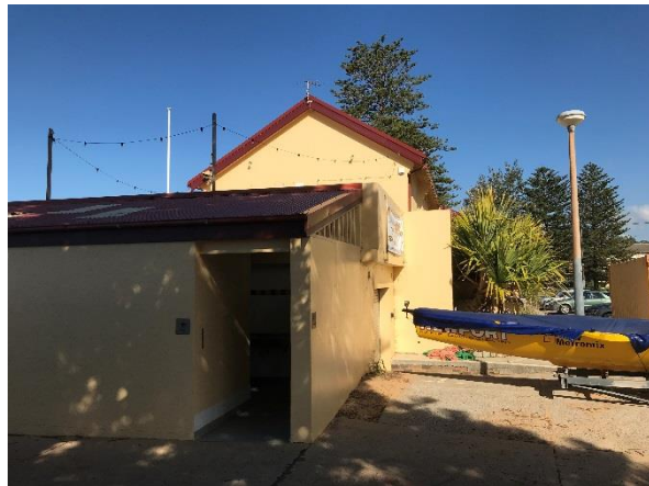
Figure 60. View to the entrance of the female public toilets along the northern skillion lean to. (Source: Heritage 21, 23.05.18)
