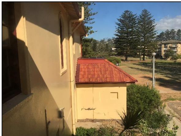
Figure 102. View of the Southern wing as seen from the office above the entry portico. (Source: Heritage 21, 23.05.18)
