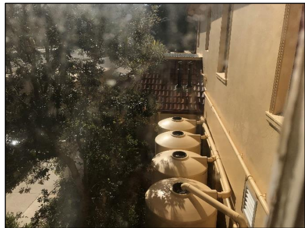
Figure 101. View to the Western elevation from a window in the office above the entry portico. Note water storage tanks and northern wing beyond. (Source: Heritage 21, 23.05.18)
