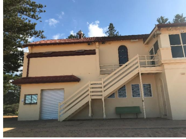
Figure 63. View of the Southern wing extension. Note the three-tiered roof extension. (Source: Heritage 21, 23.05.18)
