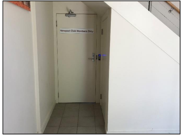
Figure 71. Restricted Access Door to main building on ground floor. (Source: Heritage 21, 23.05.18)
