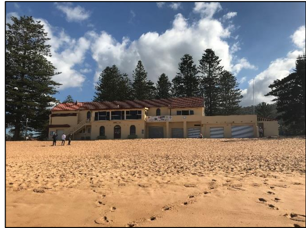
Figure 57. View of the eastern elevation as seen from Newport beach. (Source: Heritage 21, 23.05.18)
