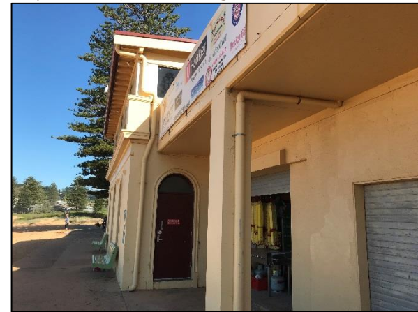
Figure 59. View of the door leading into the first aid room on ground floor and verandah extension in front of storage yards. (Source: Heritage 21, 23.05.18)
