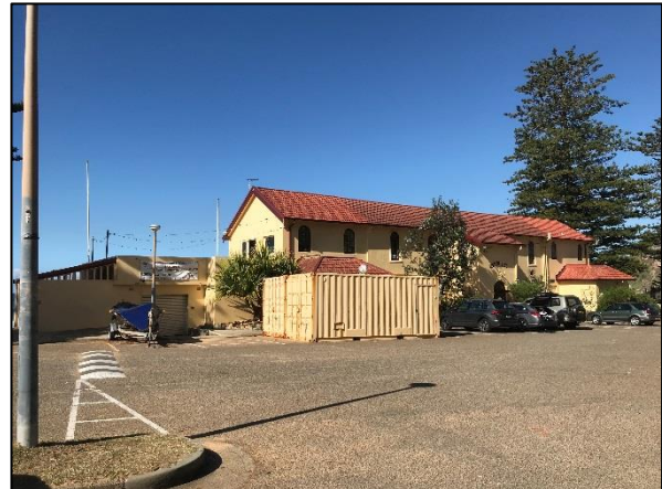
Figure 51. View from the north western corner of the parking lot looking towards the subject building. (Source: Heritage 21, 23.05.18)
