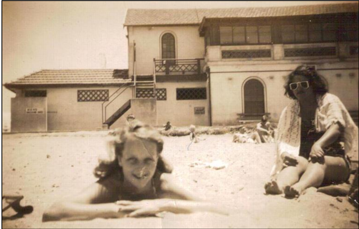
Figure 33. Image of eastern façade of the Newport Clubhouse, c. 1948. The photo shows the removal of a portion of the balustrade for the addition of emergency stairs. 'Ann Kristensen on sand at Newport Beach'. 83
