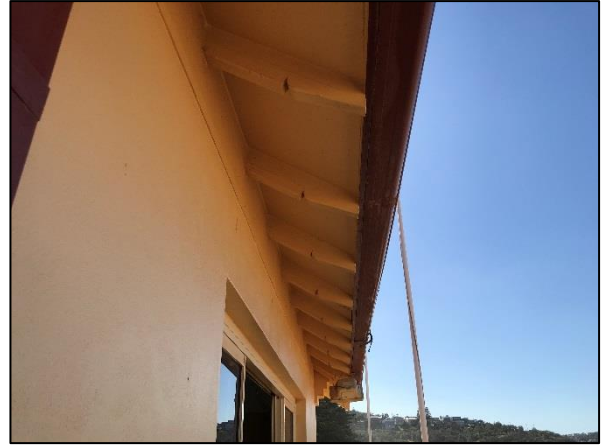
Figure 105. Note timber batons along roof line of original building in the centre. (Source: Heritage 21, 23.05.18)
