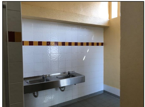
Figure 81. Female public Toilets (Source: Heritage 21, 23.05.18)
