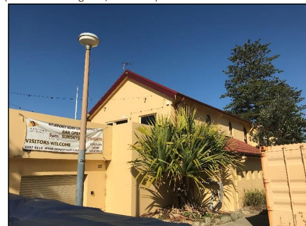
Figure 61. View of the hotel from the north-west corner of the subject building. (Source: Heritage 21, 23.05.18)
