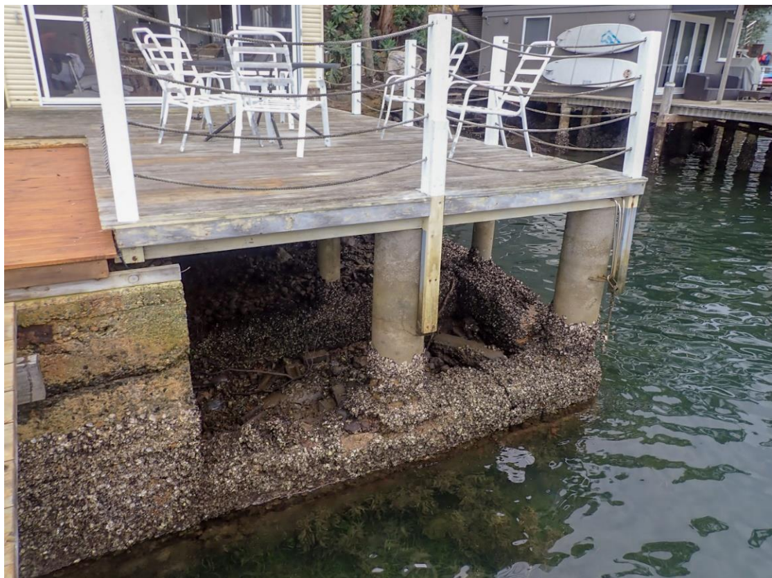
Photo 4. The section of timber decking to be removed to allow for installation of a new mesh skid.
