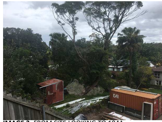
IMAGE 3: FROM SITE LOOKING TO 104A
