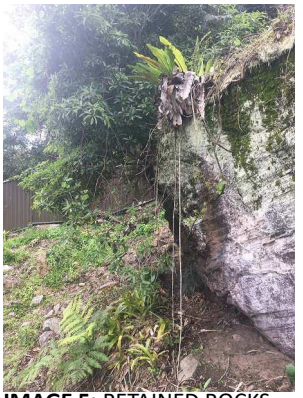
IMAGE 5: RETAINED ROCKS ON SITE
