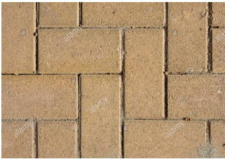
Existing brick paving
