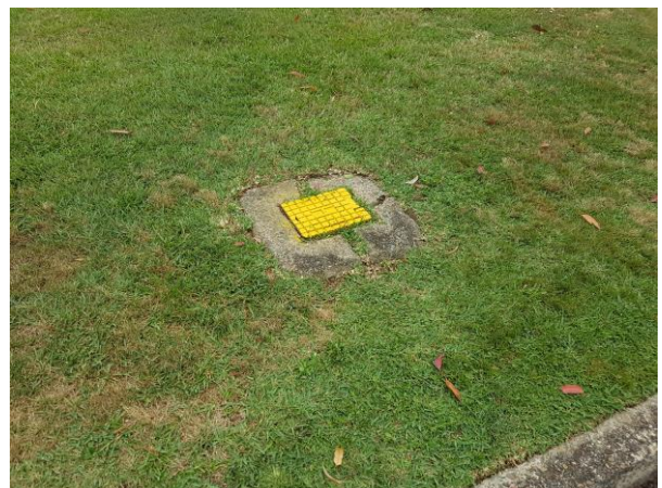
Reticulated water hydrant in pathway
