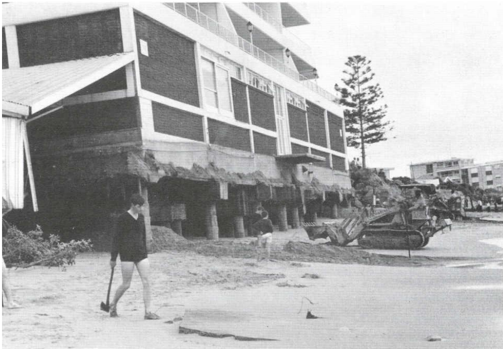
Figure 6: Exposure of Flight Deck foundations and damage to surrounding areas on 4 September 1967, as a result of a coastal storm (from Public Works Department [PWD], 1985)
