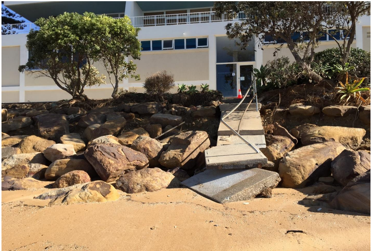
Figure 4: Damaged beach access path and revetment at Flight Deck on 23 June 2016
