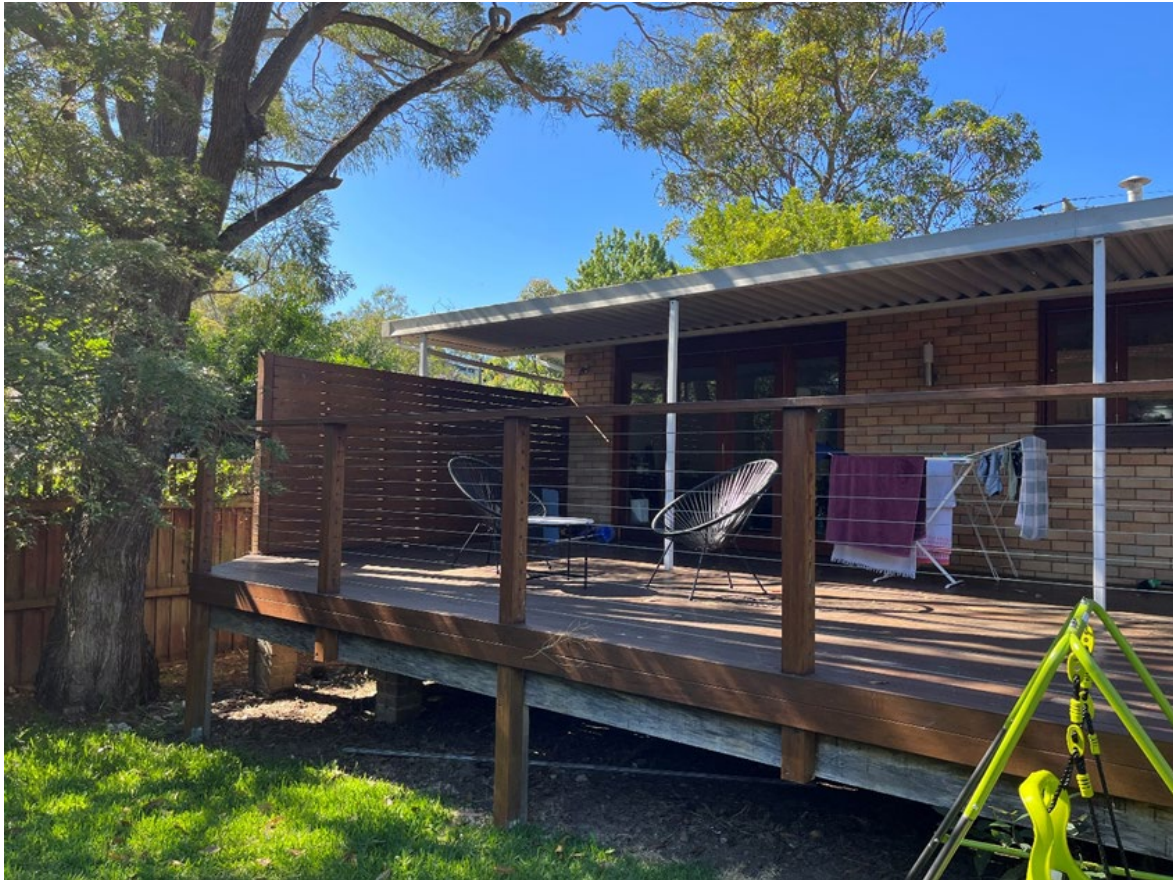
Image 4 – Existing rear timber deck, screen and metal awning
