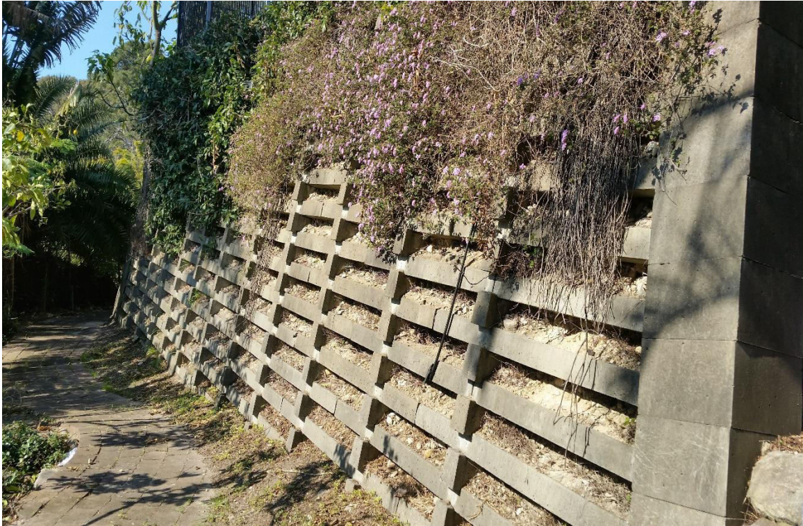
Pre-cast concrete crib retaining wall
