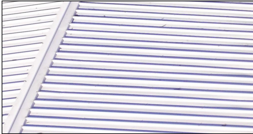
(3) METAL COLOURBOND ROOFING - COLOUR TO MATCH EXISTING
