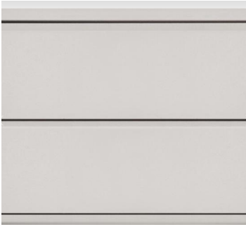
Weathertex Cladding - To Match Existing
