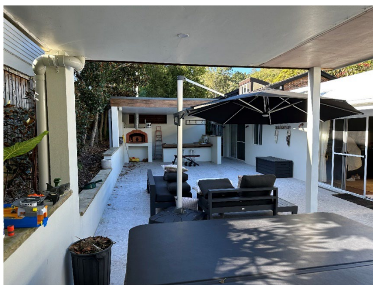
FIGURE 2 – Existing alfresco area at the rear of dwelling.
