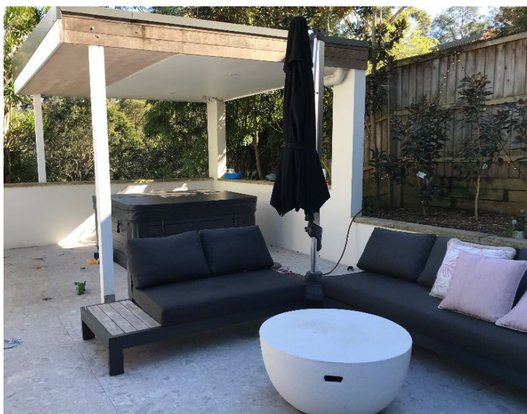
Figure 8 – Existing structure to be removed and replaced with the swimming pool.
