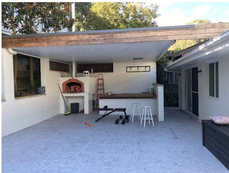
Figure 7 – Existing structure to be enclosed to create cabana.
