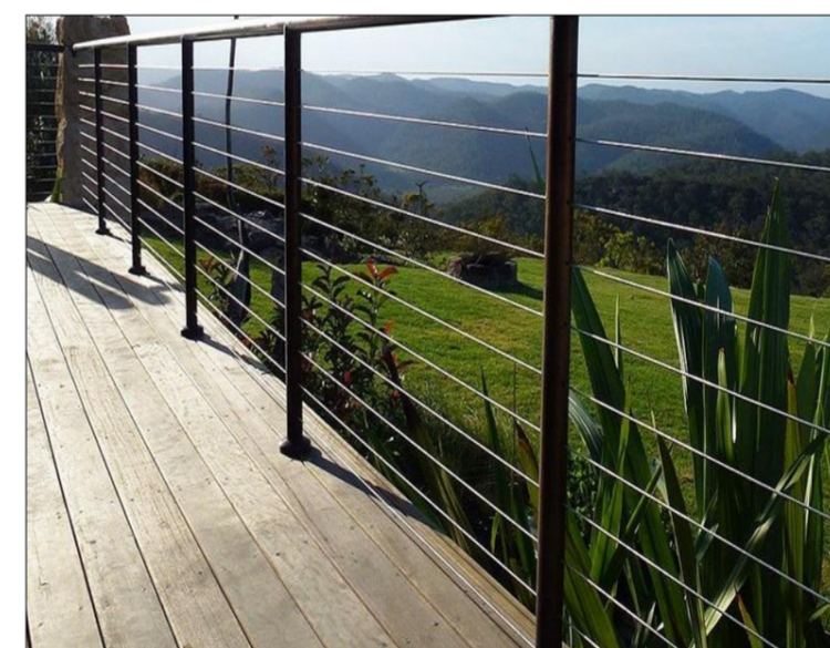
all balustrades rendered blockwork steel wire balustrade
