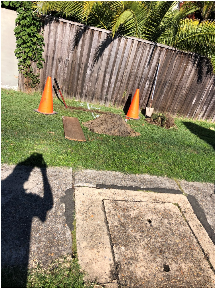
Figure 1.3 Stormwater pipe Pothole
