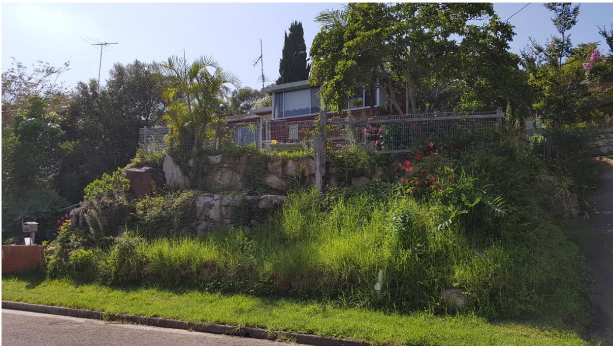
Front view of the dwelling – exposure of rock outcrops and rock wall
