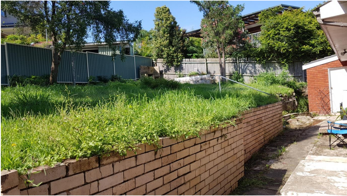
Backyard of the dwelling - exposer of rock at the right corner
