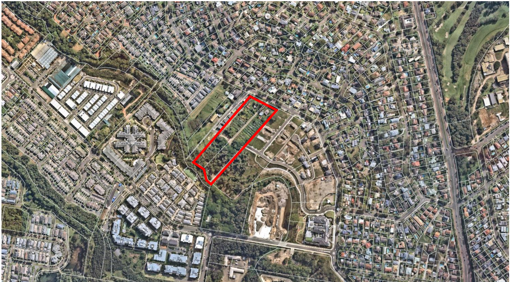
Locality photo showing the location of 43, 45 and 49 Warriewood Road, Warriewood (to accompany Form A - Request for the Planning Secretary's Requirements)
