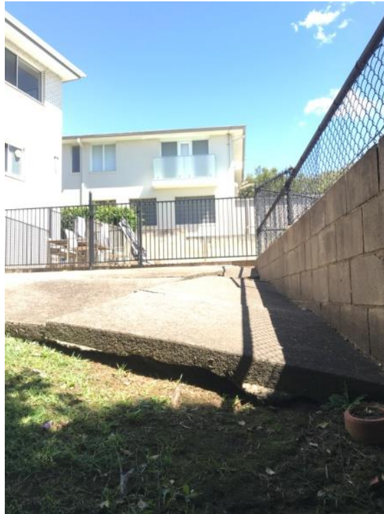
Photograph 4: Subsidence of the concrete slab at No.10
