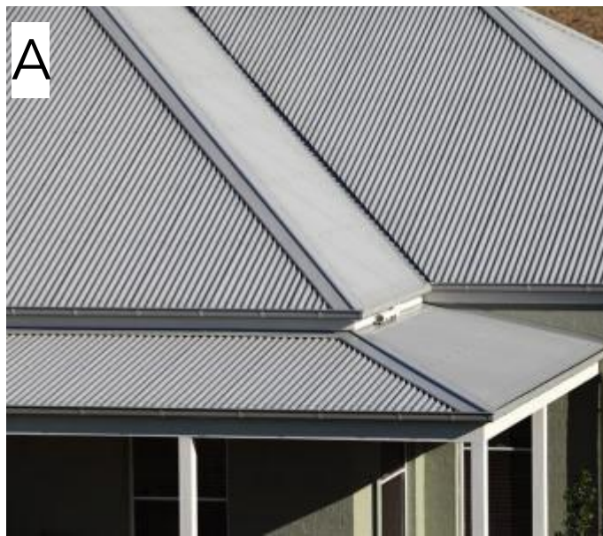
NEW METAL CLAD ROOF MED - DARK COLOUR TO OWNER'S REQUIREMENTS
