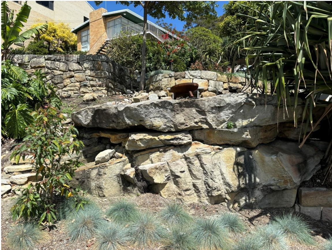
Photograph 5: View of outcropping fractured bedrock within the southeastern corner of No.74
