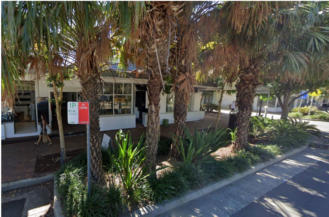
Photograph 1: View of subject site fronting Barrenjoey Road
