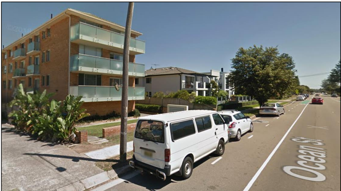
Figure 4 – Adjoining residential flat building located to the north of the site along Ocean Street.
