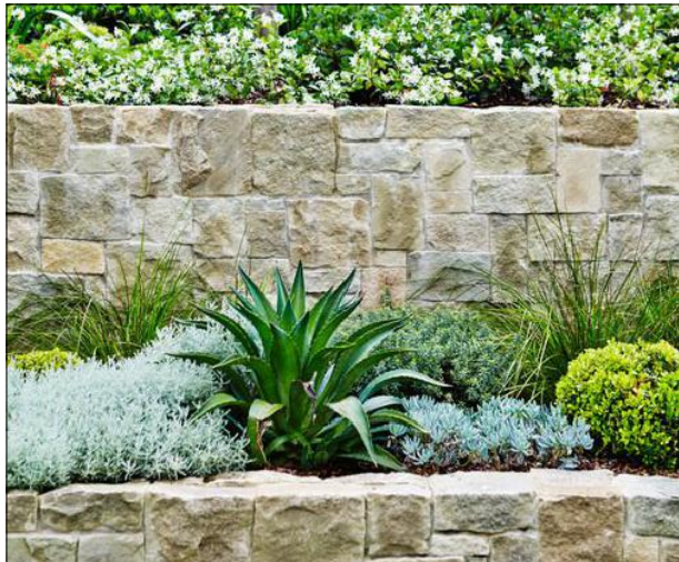
E08 SANDSTONE BOUNDARY WALL
