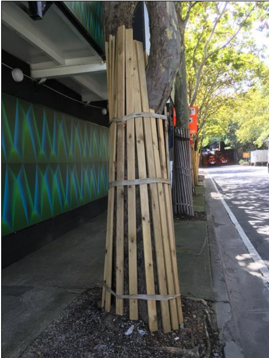
Figure 10. Stem protection measures established in the City of Sydney Council.
