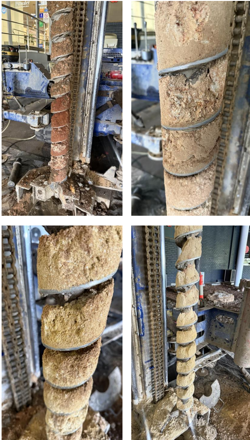
Photo 2 – Subsurface soil samples retrieved from the boreholes during the investigation
