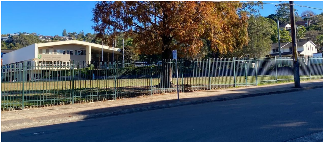
Figure 6 Existing 2.2m iron fencing located at the school boundary on Alfred Road
