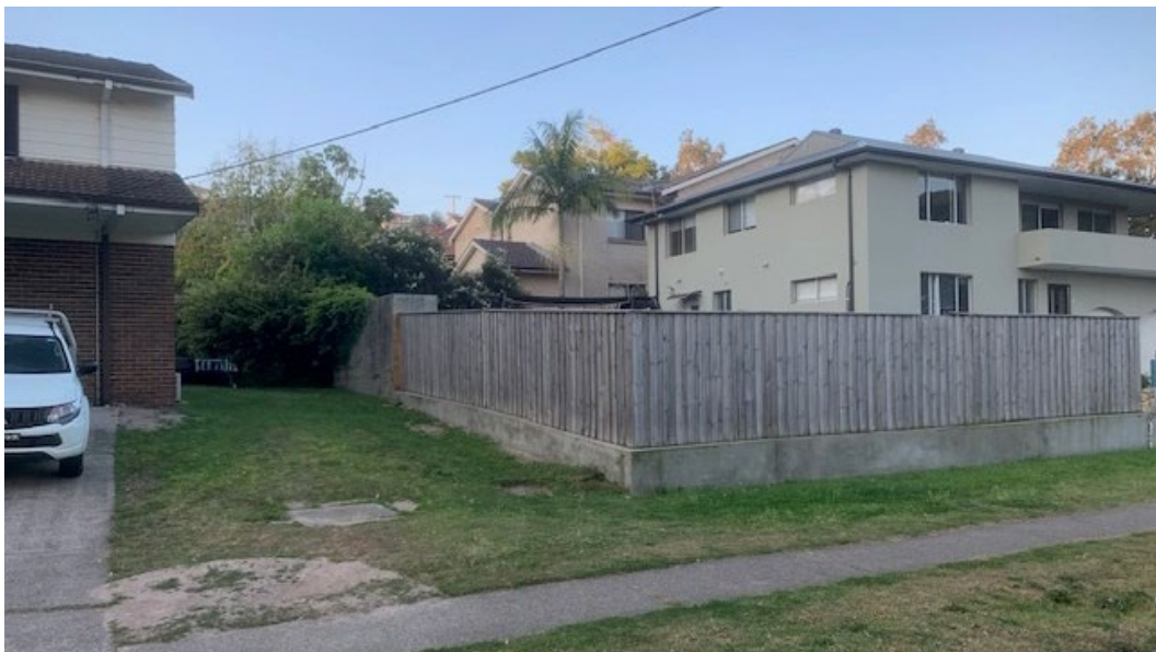
Figure 7 Existing fencing at 42 Alfred Road along the Federal Parade Boundary
