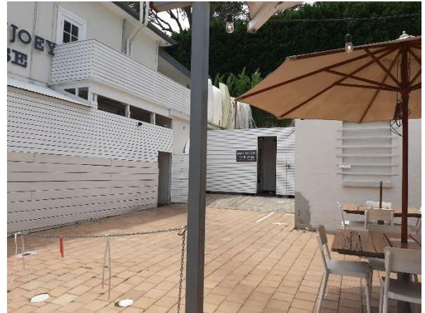
Figure 5 –Rear dining area with Barrenjoey House visible on the left.
