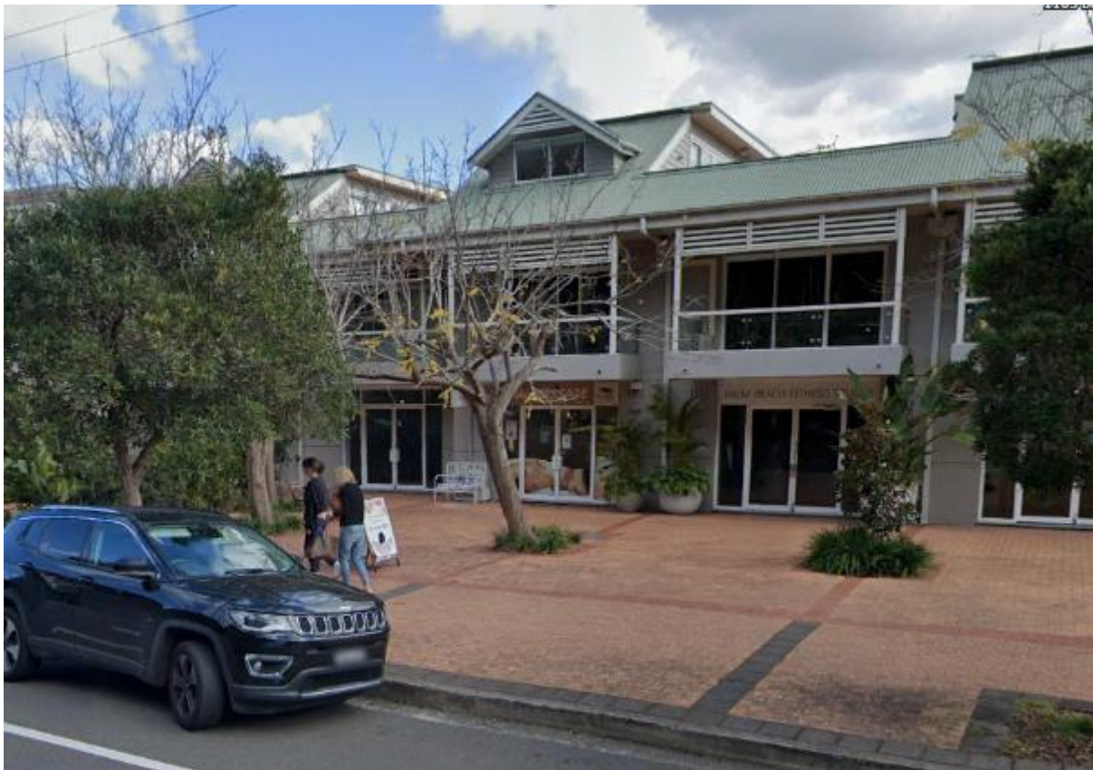
Figure 3 – Photograph of the existing 3 storey mixed use development located on the subject allotment
