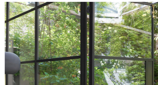
F07 : CLEAR GLASS WITH POWDERCOATED ALUM. FRAME EQ. DULUX COLORBOND MONUMENT
