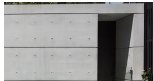
F03 : EXPOSED PRECAST CONCRETE PANEL
