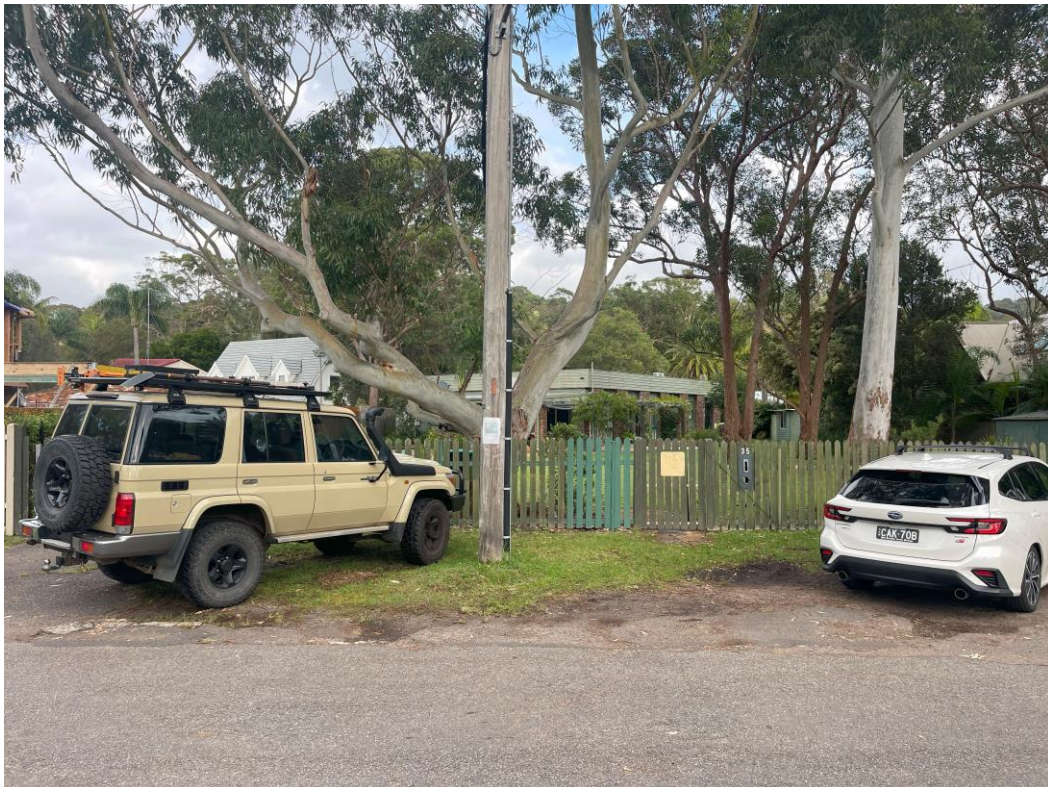
Fig 3: View of the subject building, looking south-west from John Street
